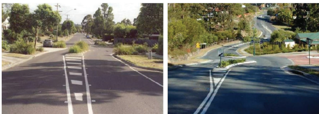
Figure 5.4.5.2: Examples of modified T-intersection channelisation.
