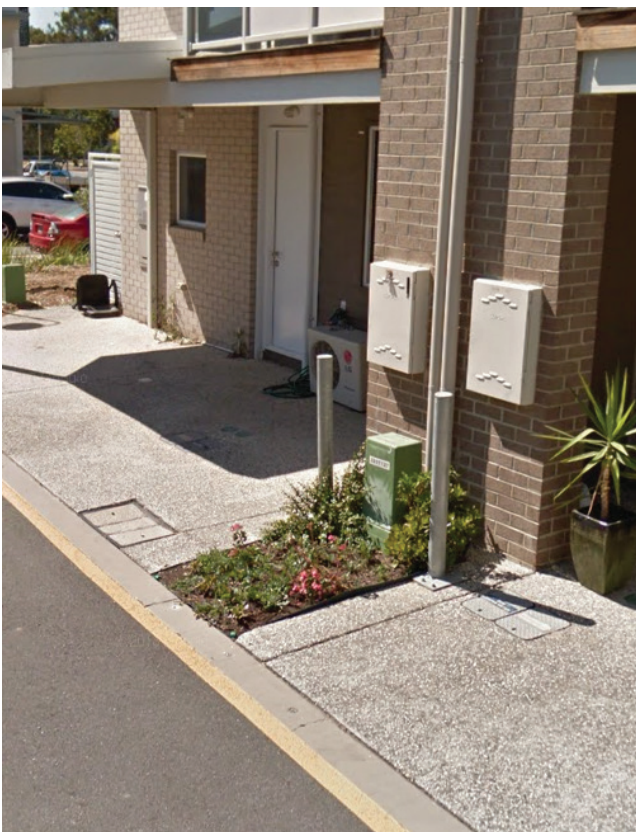
Figure 6.1.3 Laneway electrical service pillar with bollard protection
