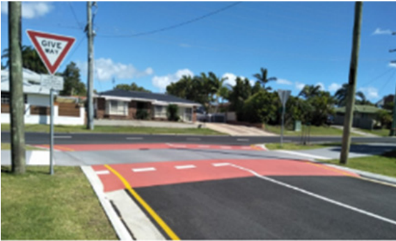
Figure 2.2.2 - Example Crossing Treatment – Raised priority Crossing
