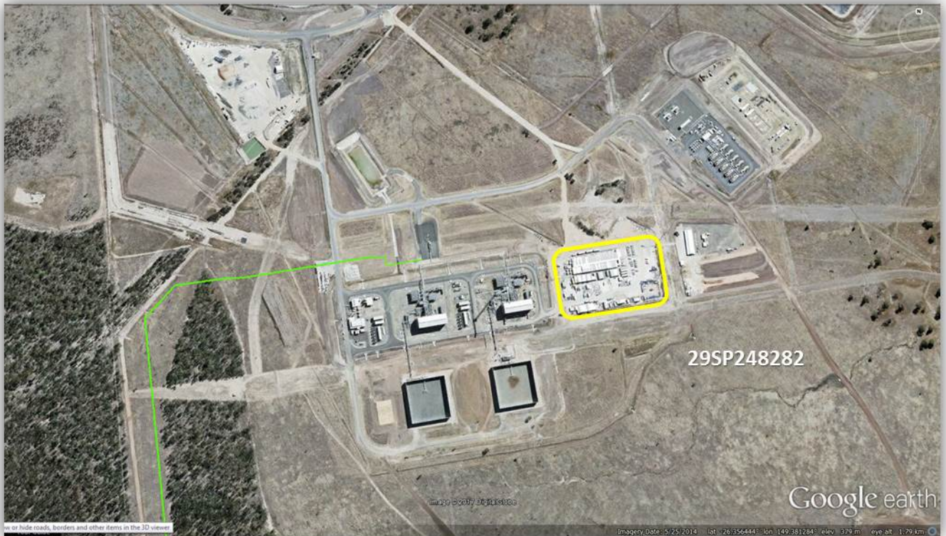
Figure 5 : Location of Laydown at Reedy Creek
