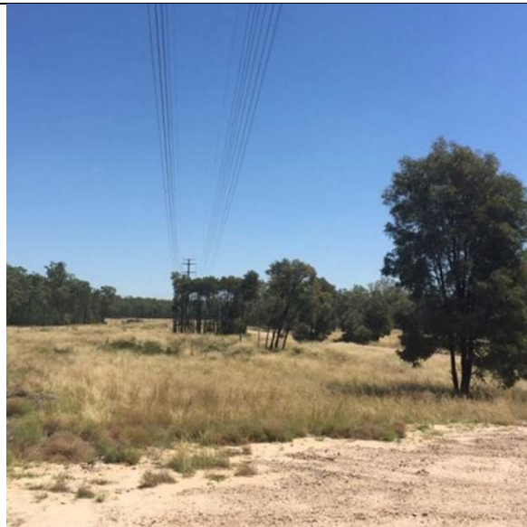
Plate 2 – Example of 132kV overhead transmission line RoW with selective clearing and grass left undisturbed.
