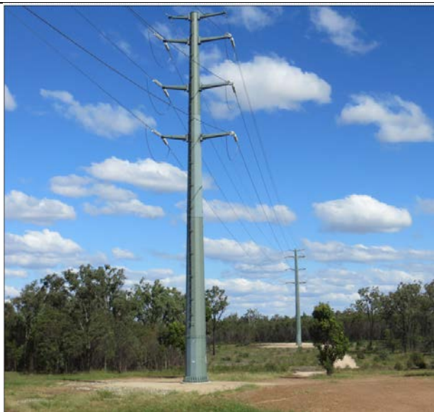
Plate 1 – Example of 132kV overhead transmission line RoW and pad.
