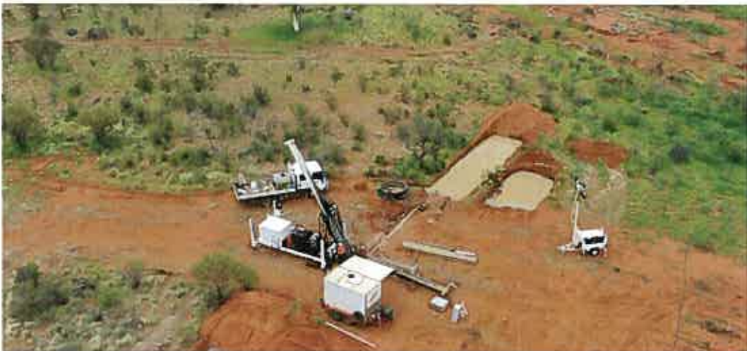
Plate 2 – Typical diamond drill site layout (site in existing disturbed area)
