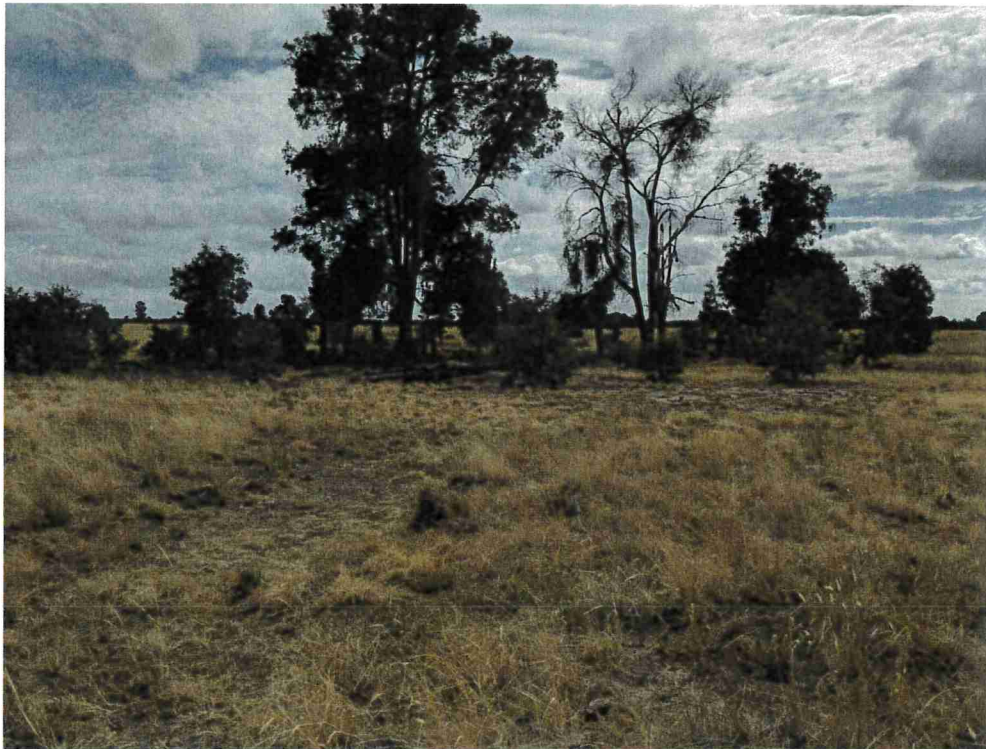
Photo 3 – Abandoned and partially demolished cattle yards
