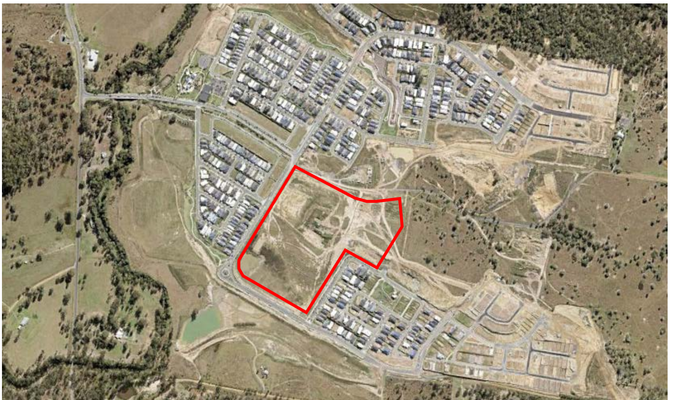
Figure 2. Aerial of Proposed School Site
