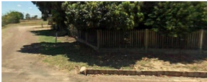
Figure 4 - Kerb and channel adjacent to the rear laneway access indicated above.
