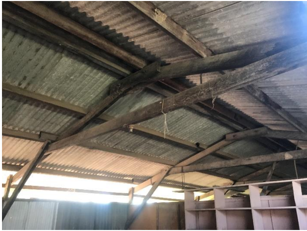
Bolted timber frames supporting roof purlins and wall girts are positioned at 2.7m centers along the length of the building.
