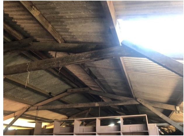
Bolted timber frames supporting roof purlins and wall girts are positioned at 2.7m centers along the length of the building.
