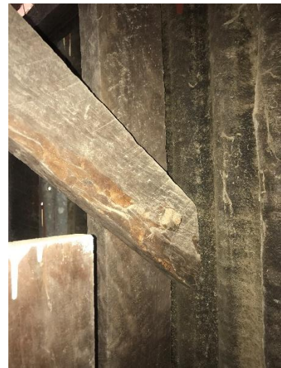
Bolted timber frames supporting roof purlins and wall girts are positioned at 2.7m centers along the length of the building.
