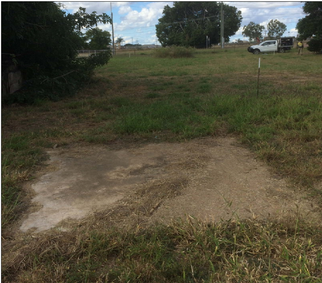
Figure 4: Pre-existing concrete slabs, located in the centre of the site. Photo looking east
