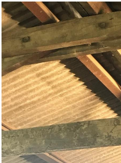
The main building frame has bolted connections, forming a braced frame.
