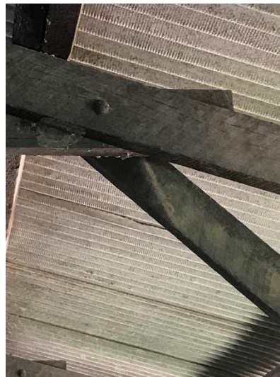
The main building frame has bolted connections, forming a braced frame.
