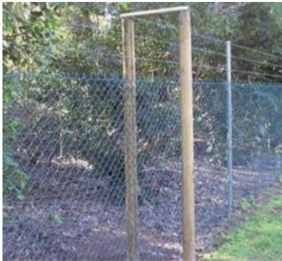
Plate 1 - example wooden bridge over security fencing designed to facilitate the safe movement over the fence (source: Koala-sensitive Design Guidelines, DES 2022)
