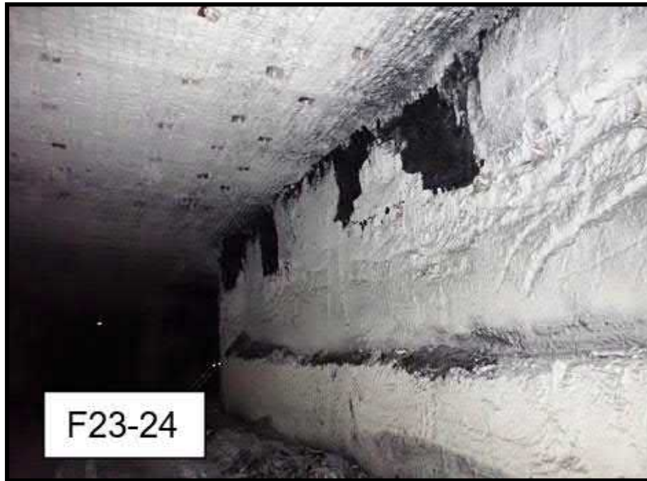
Figure 38. Typical Thin Rib Spall at Ensham after Secondary Coal Recovery – F23-24, 109A Panel
