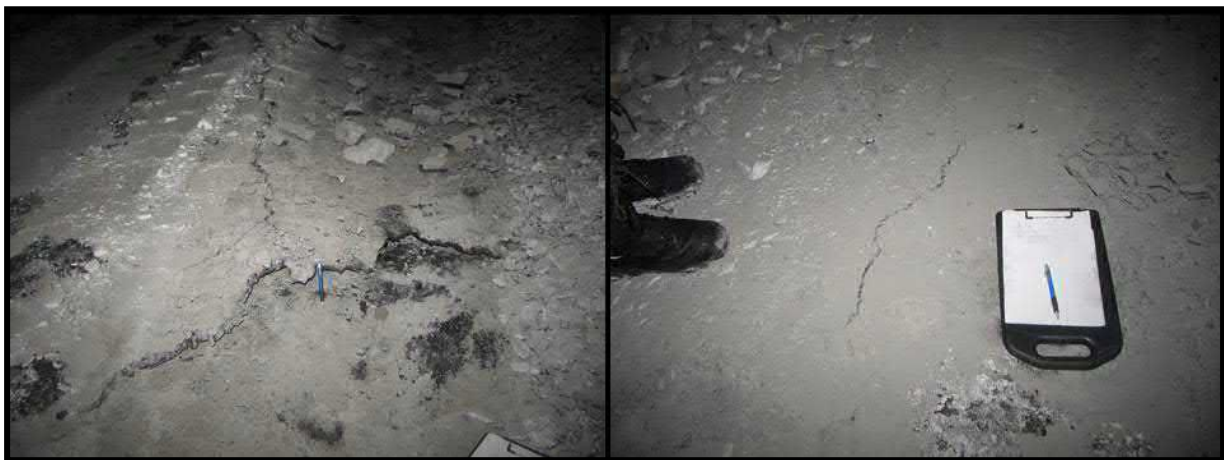
Figure 43. Minor Cracking of the Coal Floor, 101 Panel
