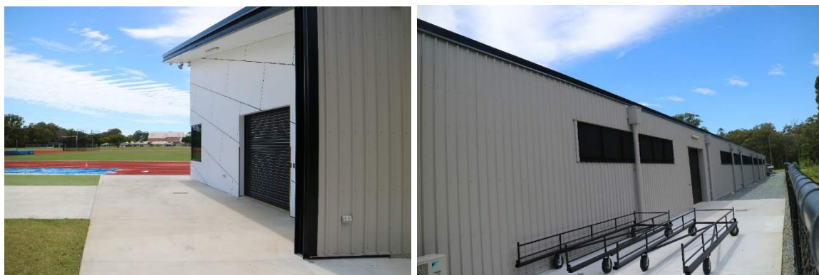
Figure 7 The existing structure is a grandstand, with constructed of ColorBond Steel.
