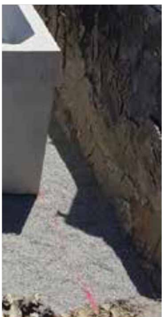
ALIGN TANK WITH SETOUT LINE
