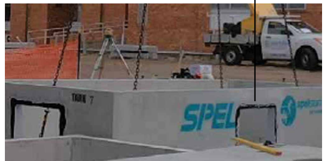
PREPARING TO SKIM A TANK INTO PLACE
