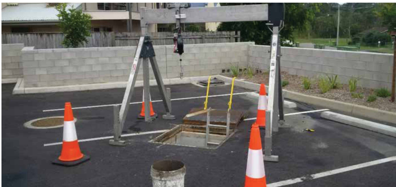
FIGURE 4 AtlanFilter install set-up
