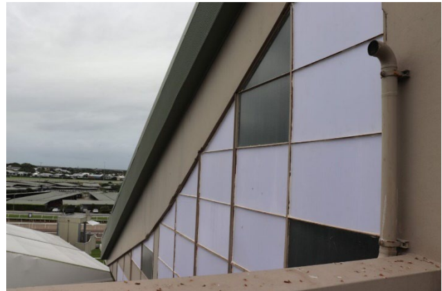
Picture 6 Roof and panels closing in the upper tier
