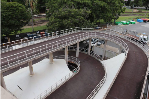
Picture 7 Semi-circular ramp, with circular beams and asphalt overlays
