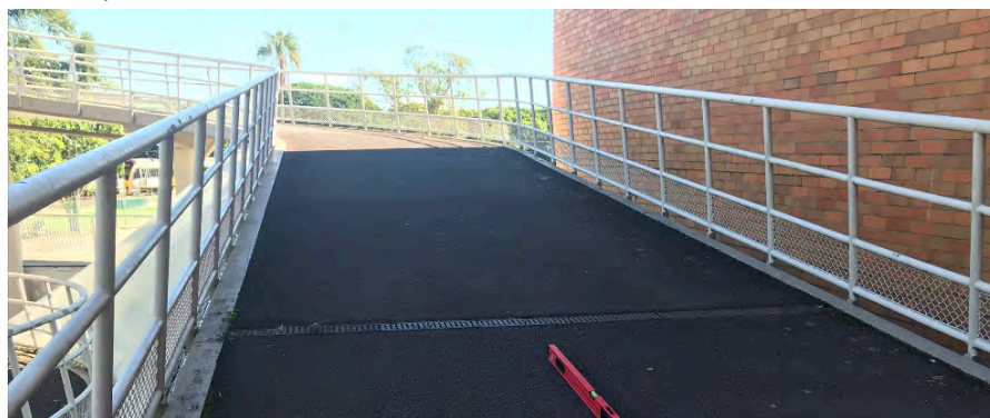
Compliant handrail arrangement below from AS1428.1-2009
