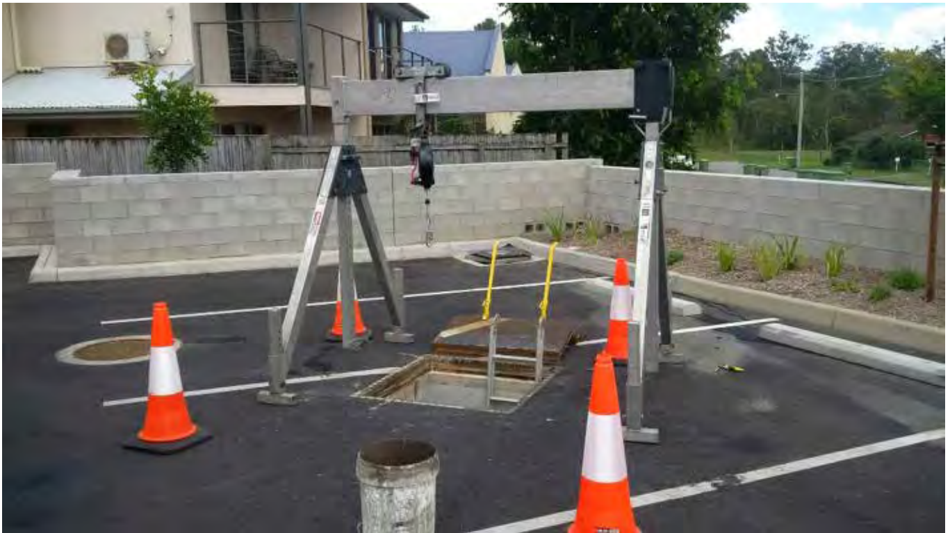
Figure 4. SPEL Filter install set-up
