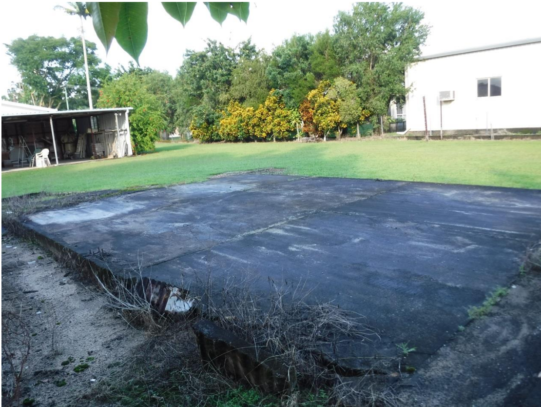
Photo 1 – 5 Ryrie St, El Arish
