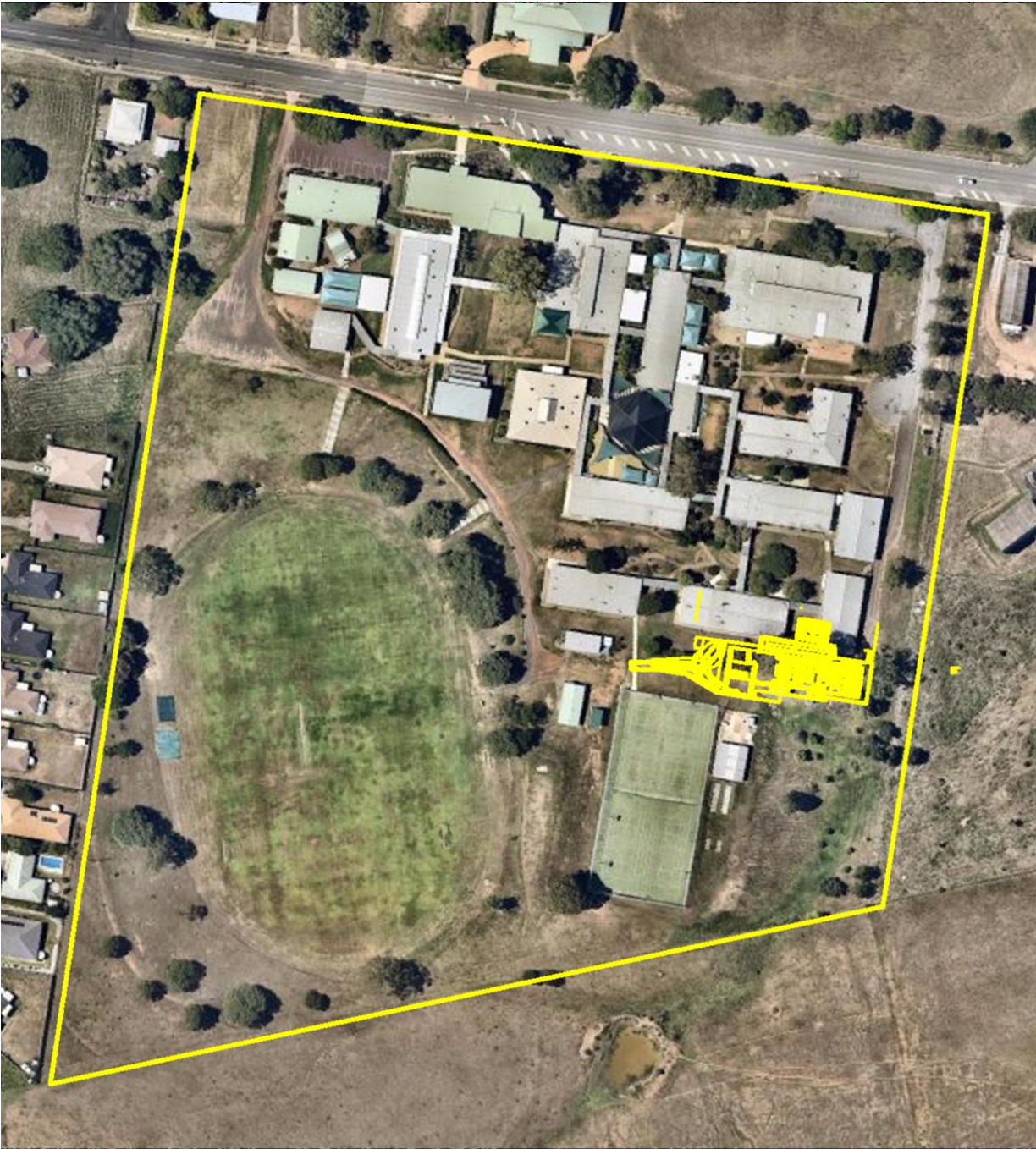
Figure 2 - Aerial View of Existing Site
