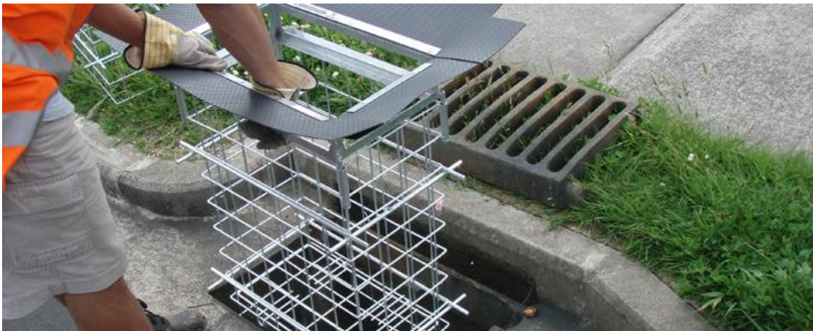
Figure 7-3 EXAMPLE FILTER BASKET 1
