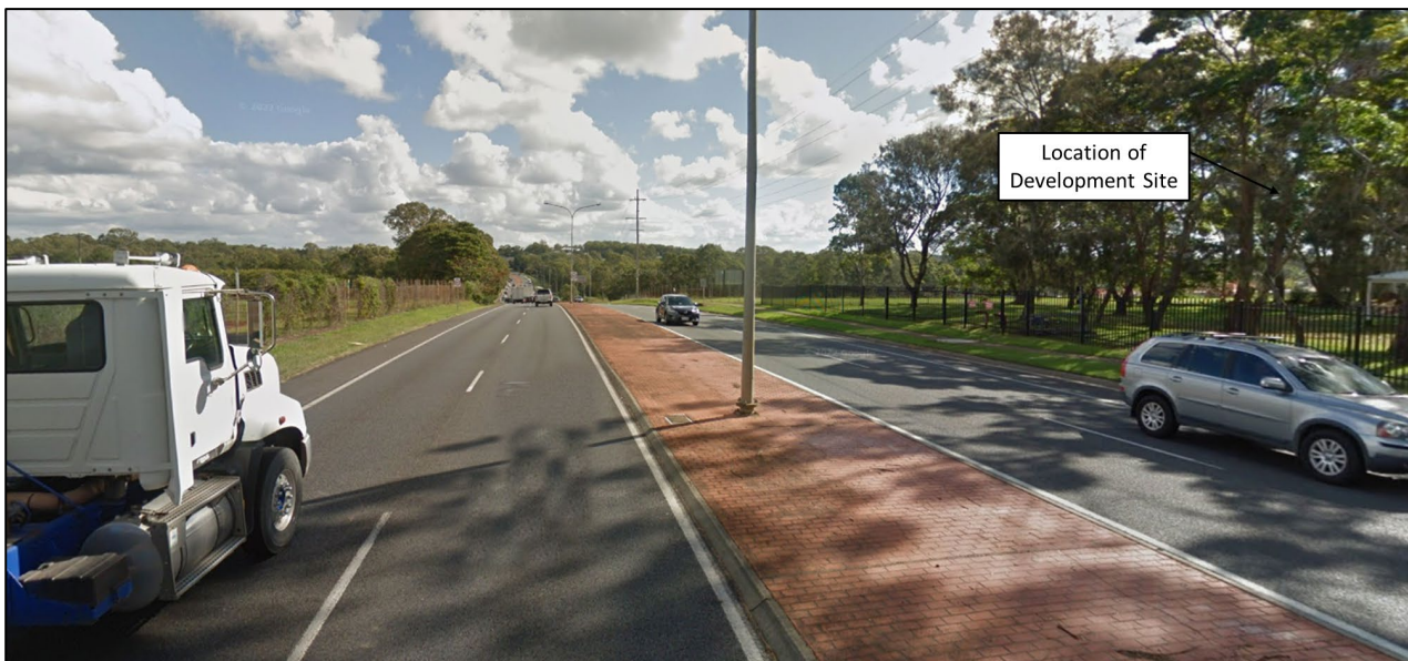
Figure 2-2 Finucane Road (Facing west)
